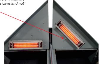
UniHeater is mounted with brackets facing the cave as well. There is an angle on the dish inside UniHeater, this provides a better dispersion of heat in the cave. When you installed correctly.
